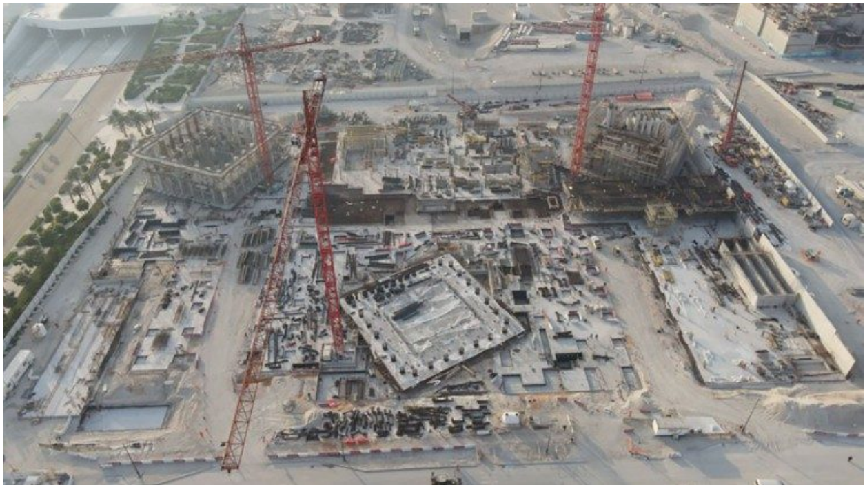
Abrahamic Family House (under construction)
